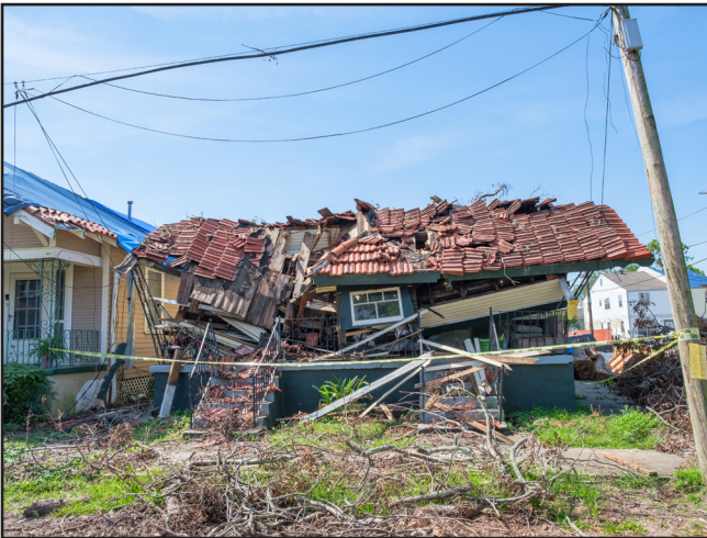
A house damaged by Hurricane Ida in New Orleans on Oct. 9, 2021.
